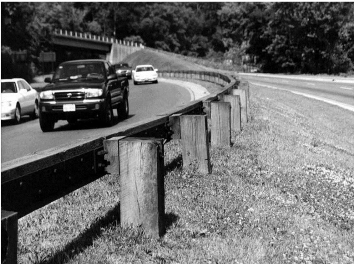
**Figure** Steel-Backed Timber Guardrail
