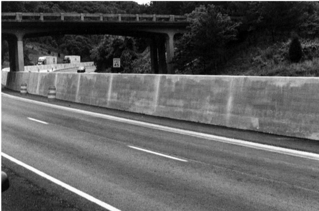
**Figure 15.7** Single-Slope Concrete Median Barrier
