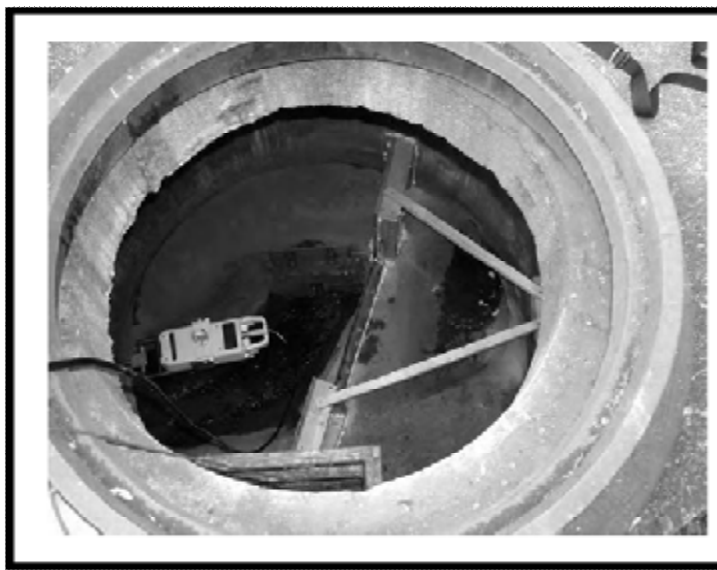
Fig (11) Flow meter and weir installation in a manhole for monitoring incoming and outgoing flows.
