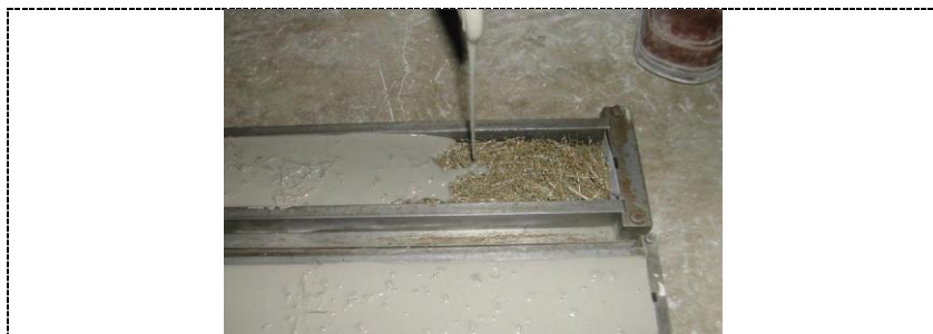
Figure 1: Casting procedure of SIFCON [12].
